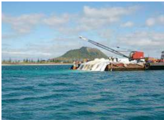
Figure 4.15: Construction of Multi-Purpose reef (Source: ARS Marine Consultants). (a) Design of the Reef, (b) Attaching geotextile containers to the web, (c) winching reef to the seabed, (d) filling geotextile containers with sand.
