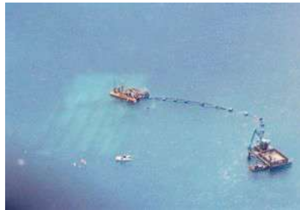
Figure 4.15: Construction of Multi-Purpose reef (Source: ARS Marine Consultants). (a) Design of the Reef, (b) Attaching geotextile containers to the web, (c) winching reef to the seabed, (d) filling geotextile containers with sand.
